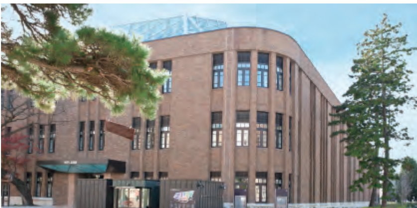
The new WPI-AIMR Main Building
